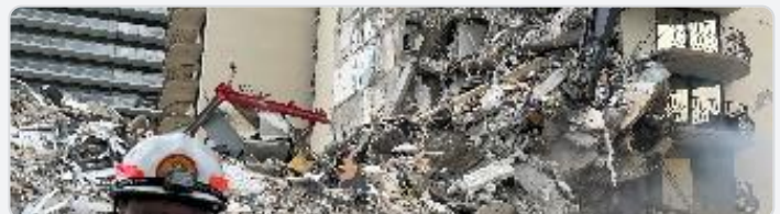
Surfside Collapse (2021) — coordinating hazard mitigation
