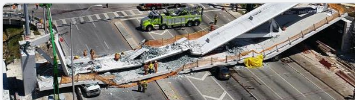
FIU Bridge Collapse (2018) — emergency response & recovery
